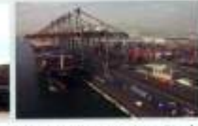
Reconstruction Project Berth No. 5-10 at Karachi Port
