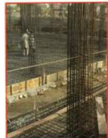
ASTM 615 Grade 60 supplied to DHO Hospital, Khairpur
