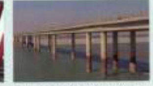
Hyderabad By Pass Bridge
